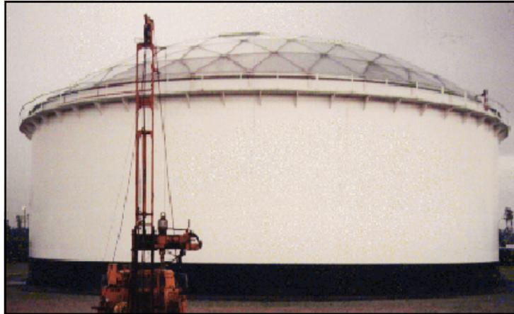
**RG-2400® AK** is a non-curing solution to tank base corrosion issues where the tank 'chime' is accessible and subject to wet/dry, chloride crevice environments where corrosion is a problem.
