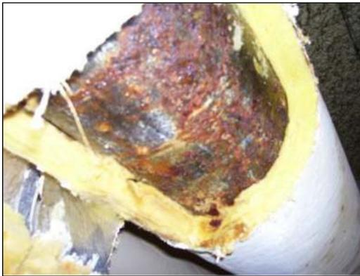
**RG-CHW** helps prevent corrosion and helps stop existing corrosion from advancing. It requires minimal surface preparation on corroded surfaces (SSPC-SP-2, Hand Tool Cleaning), which drastically reduces the overall cost of a system remediation without pipe replacement. (Integrity testing is recommended on corroded pipe).
