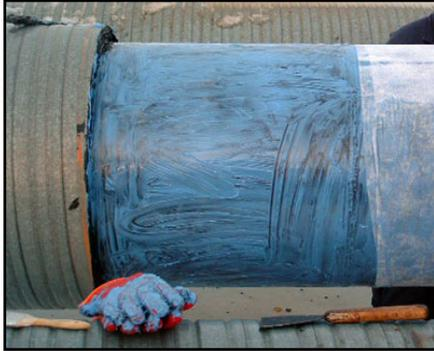
**RG-2400 ET** is a surface conversion compound utilizing mineralization technology, or the "science of Minetics"; this compound replaces the corrosion process with a mineral formation on and into the metal creating a mineral barrier 50-200 angstroms deep into the metal surface and as time passes, the mineral layer on top of the metal increases in thickness.
