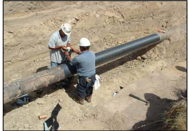
INSTALLING OUTERWRAP
