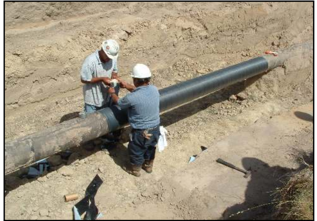
INSTALLING OUTERWRAP
