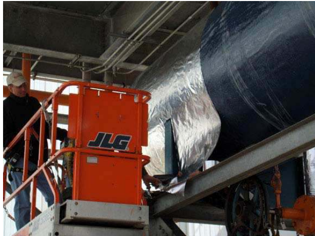
AlumaWrap™ INSTALLED OVER GeoWrap™
