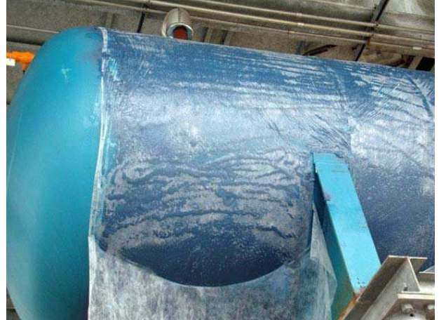
GeoWrap™ INSTALLED OVER RG
