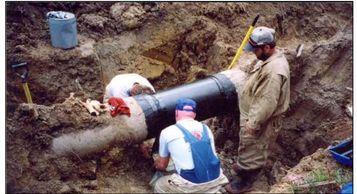
606 Filler Compound filling irregular transition areas.
