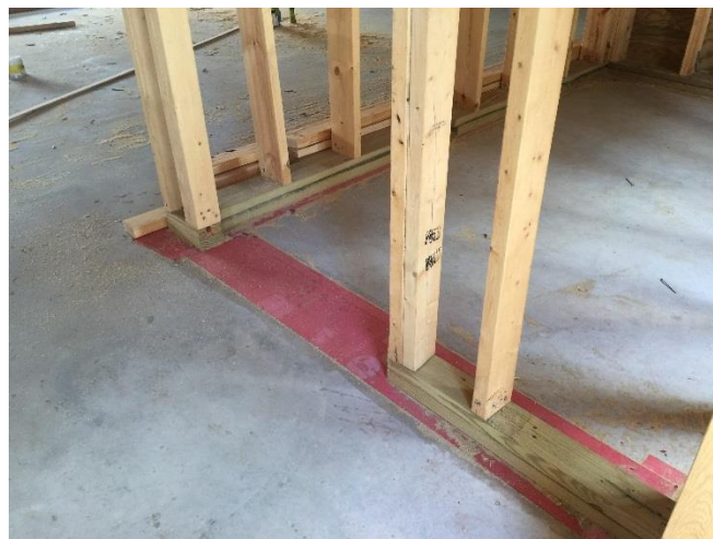
Interior sill – Orlando, FL
