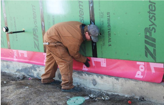
TERM Flashing Moisture|Termite Barrier installed on a residence in Ennis, TX
