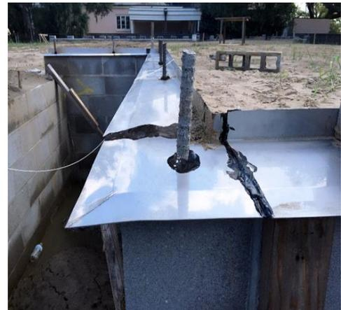
don't completely stop termites – termites can't go through the metal, but they can build their "mud tubes" around the shield. However, when they do this, the mud tube built by the termites becomes visible to pest management professionals, and can be treated.
