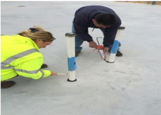
Pest management professionals know that slab penetrations are a major termite entry point. The space between the penetration and the concrete poured around it may look small, but subterranean termites can get through an opening of 0.020". Moreover, the sleeves installed on penetrations, which protect against corrosive effects of concrete, can also function as an entry tunnel for subterranean termites.
