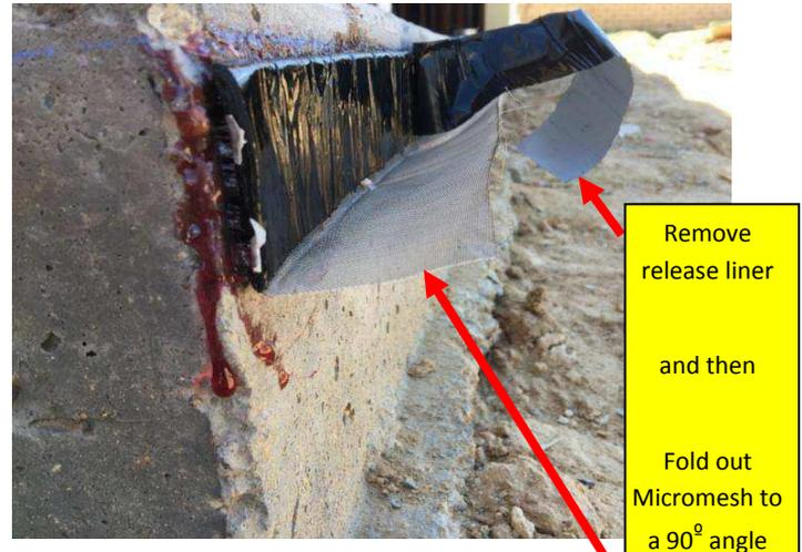
*TERM™ Isolation Joint Barrier* installed on a Waco, TX residence. The barrier is adhered to the side of the house slab. Prior to driveway pour, release liner is removed and 0.018” Micromesh screen is folded out to horizontal. The result is a barrier embed
