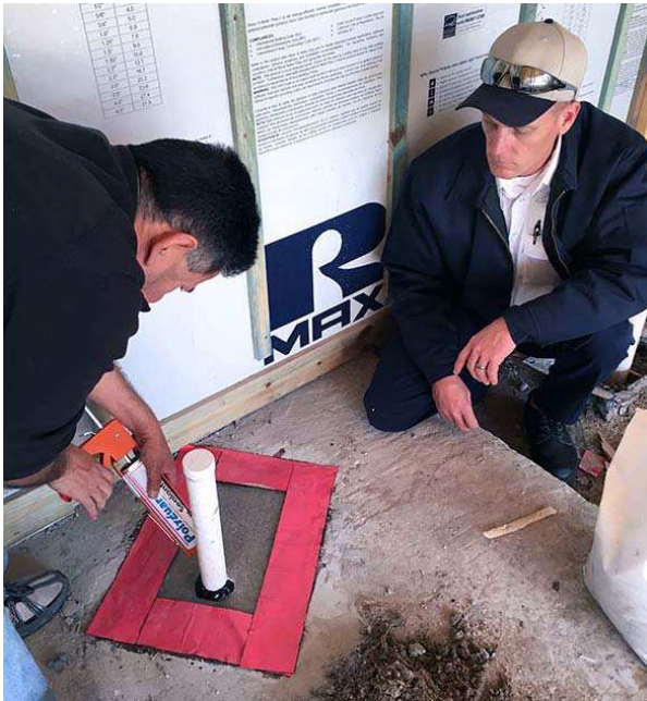
TERM All Pest Bath Trap Barrier being installed in The New American Home 2017 , an NAHB concept home to be introduced at the January 2017 International Builders Show in Orlando, FL
