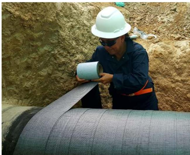
Figure 1. Installing RD-6 on a pipeline.
