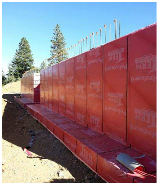
Used since 2002 to protect below grade ICF from subterranean termites Verdi, CA
