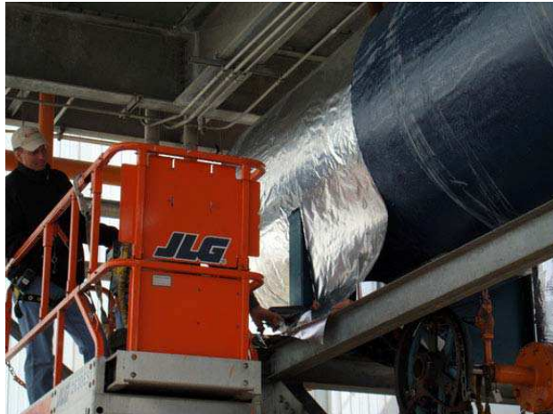
AlumaWrap™ INSTALLED OVER GeoWrap™
