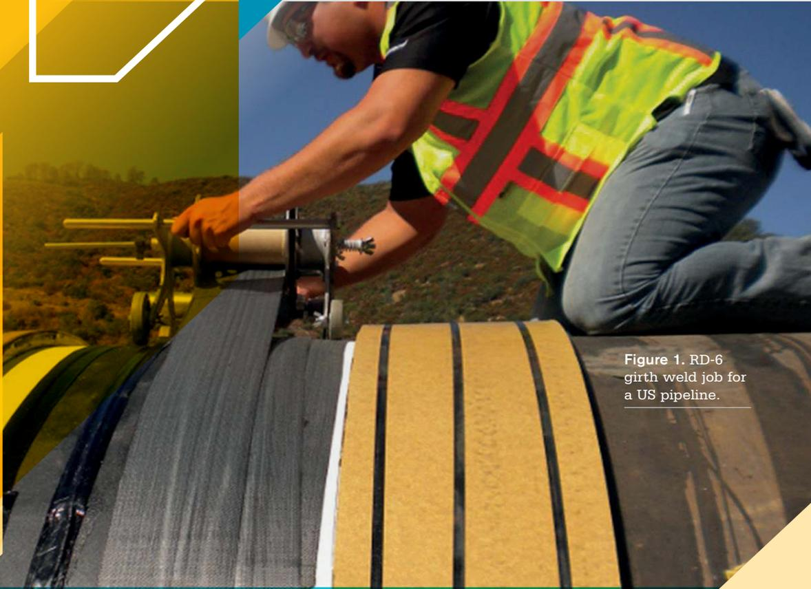
Figure 1. RD-6 girth weld job for a US pipeline.
