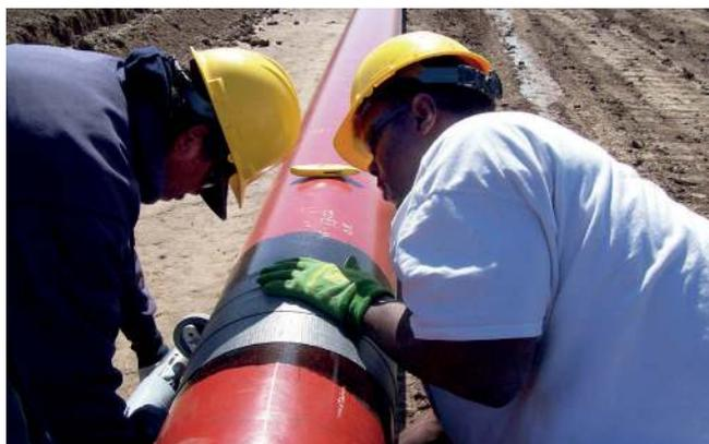
Figure 4. USA girth weld installation.
