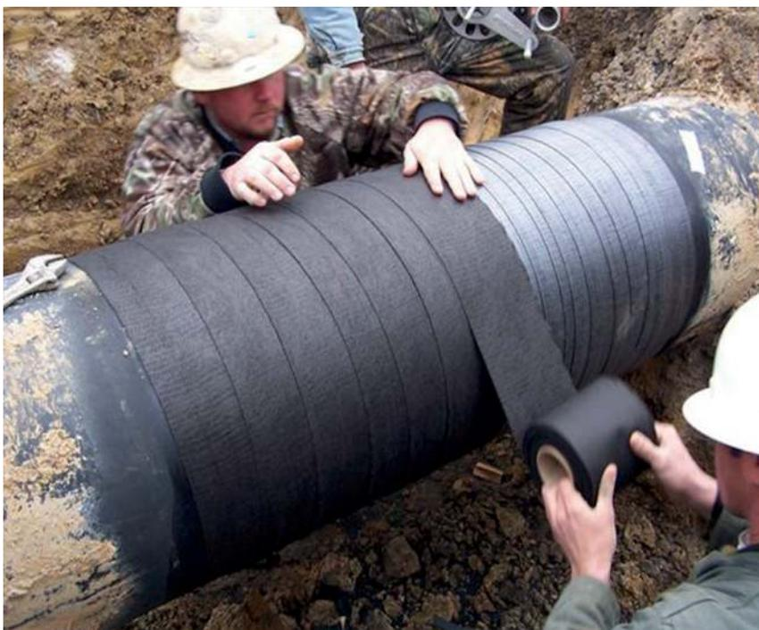
Figure 2. RD-6 rehab job in the US with SP-6 outerwrap.
